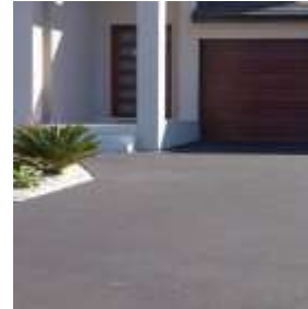
Coloured Concrete driveway
