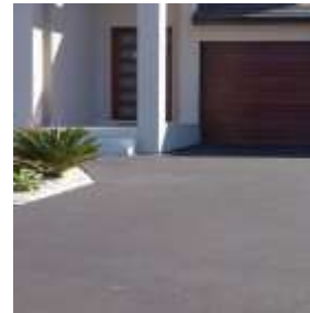
Coloured Concrete driveway
